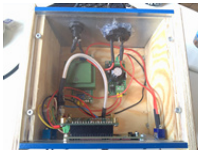
Power meter insite
